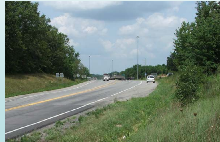
View north along US 431 to parkway interchange
