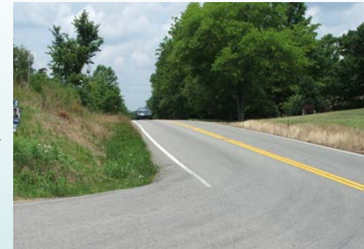
Union Ridge Road Intersection, facing north
