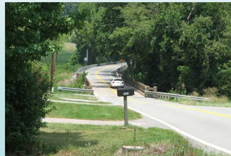
View along US 431 of southern bridge over Rocky Creek
