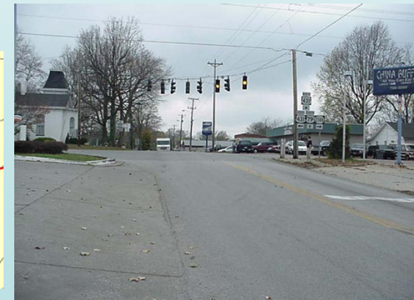
US 79 approach to intersection with US 431, facing west
