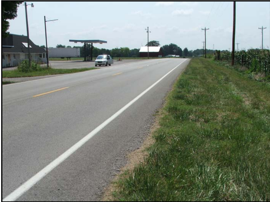
View south at Location 1-C along US 431
