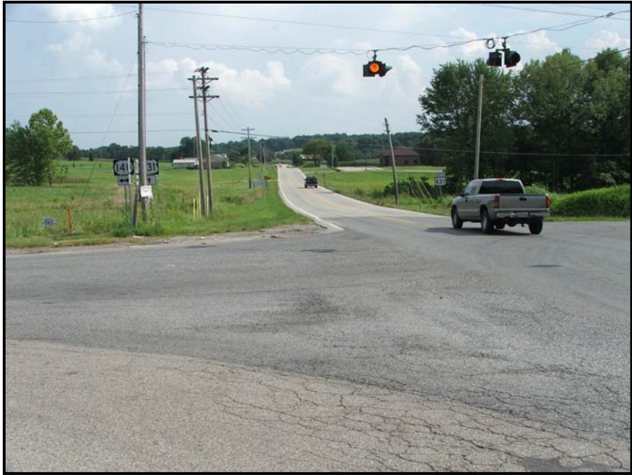
Location 2-N: KY 140 intersection with US 431, looking south, in Utica
