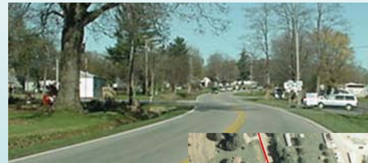
View north along US 431 at KY 250
