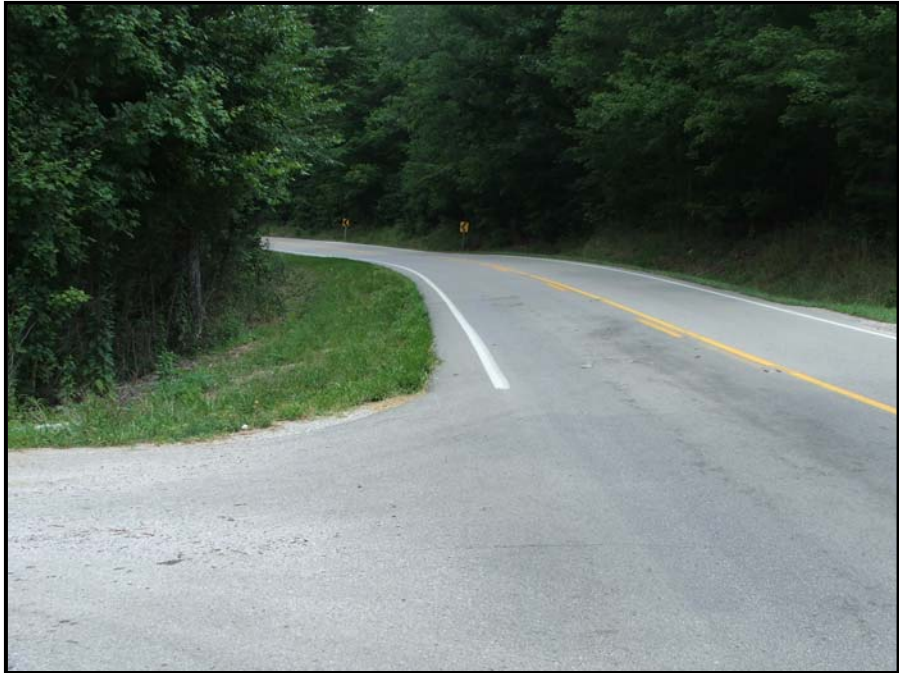
View north at Location 1-G towards a series of reverse curves north of Hollow Bill, seen from intersection with H. W. McPherson Road in Logan County
