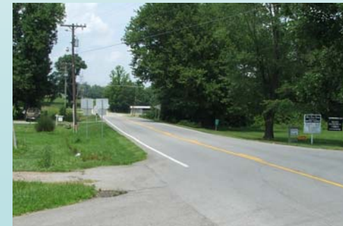
KY 2270 Intersection looking north
