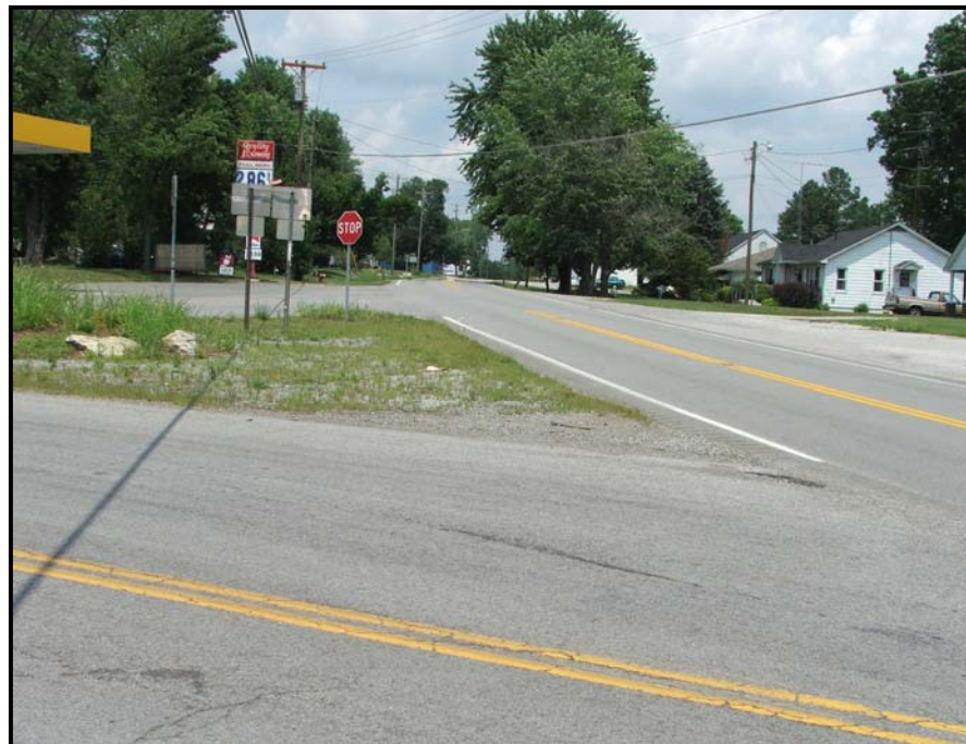
Intersection with KY 246 in Beechmont, looking north, at Location 1-O
